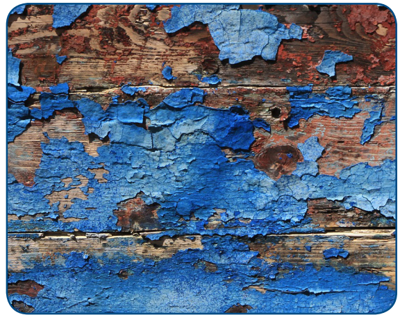
Paint containing lead was commonly used in homes built before 1978. Flaking lead paint can introduce lead into the home.
